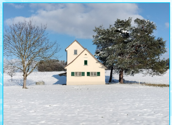
Pumpwerk in Ottikon
